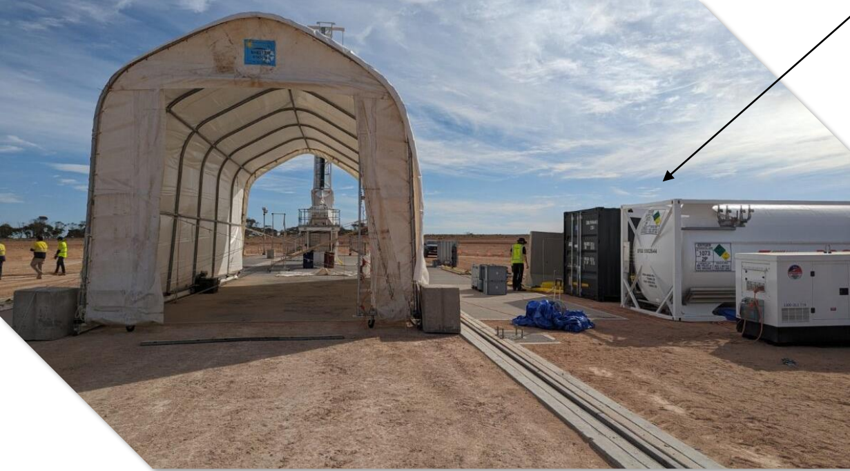
Piping and cabling – From GSE to launch rail interfaces Preparation of the rail interfaces
